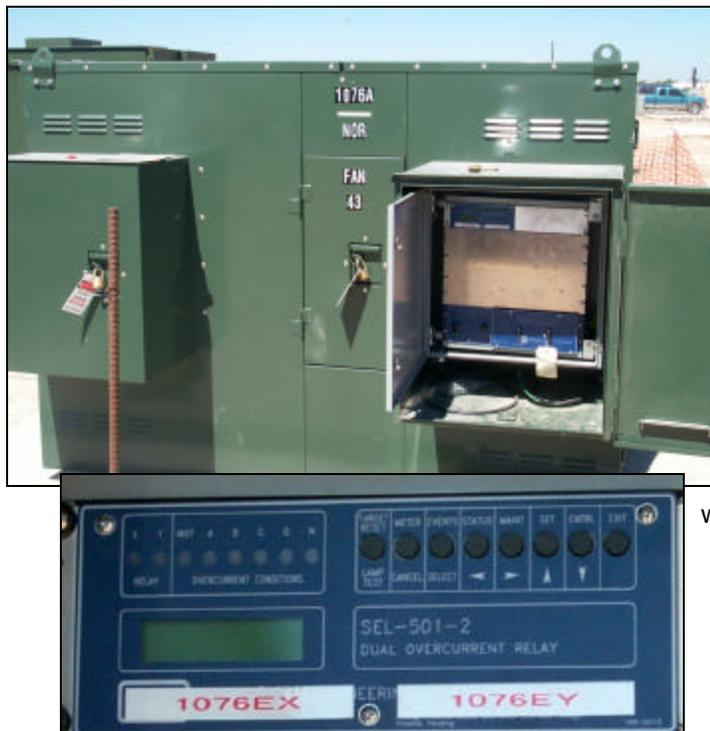
Figure 1: SEL-501-2 control in switch enclosure.
