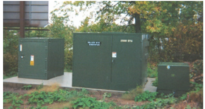
Photo shows the padmount recloser (left), three phase step-down transformer (center) and single phase transformer.
