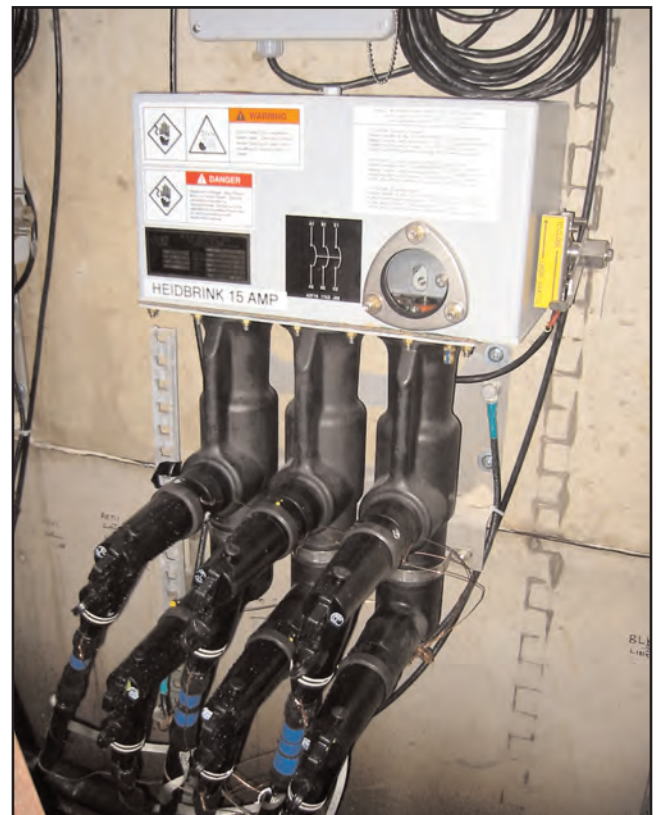
Figure 2: Three phase interrupter mounted to vault wall. Operating handle permits manual reset of all three phases and is accessible from above ground using a hookstick.
