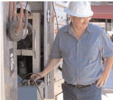
*The interrupter incorporated a top mounted motor actuator permitting above ground operation using a portable control . Future SCADA requirements can utilize the same motor actuators.*
