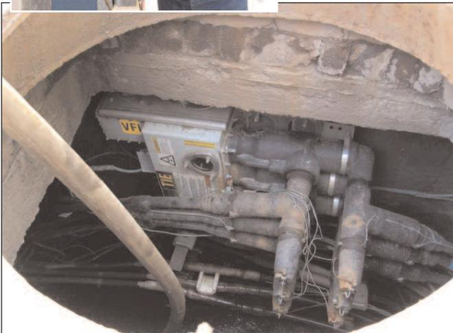
*Three phase fault interrupter mounted horizontally due to limited vault space. The vault opening is only 23" in diameter.*
