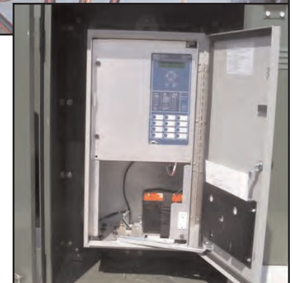
Photo above shows the recloser compartment access for cable connections.
