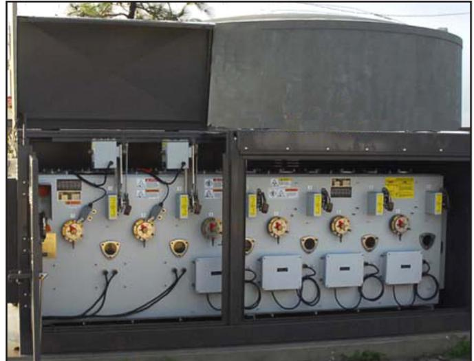
▲ Six way padmount switch with motor actuators on source ways 1 and 2.
