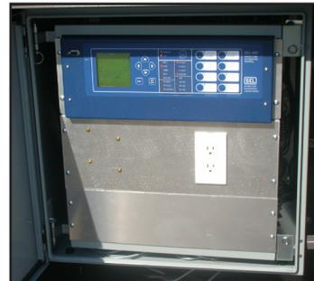
▲ The SEL 451 relay is housed in a separate enclosure on the side of the switch.
