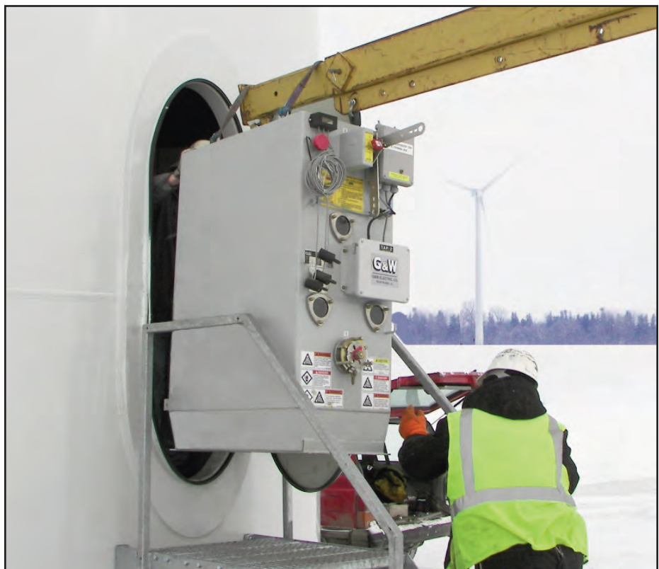
▲ Compact vertical design fits through the typical entrance opening for installation after the tower is constructed.
