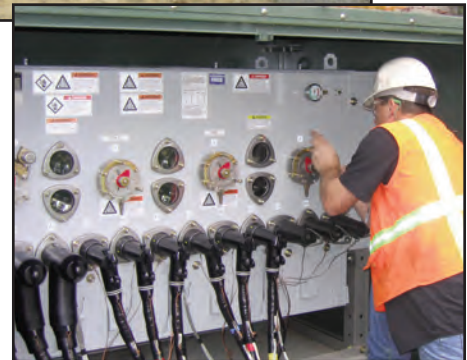
▲ Padmount switch installed outside the tower.
