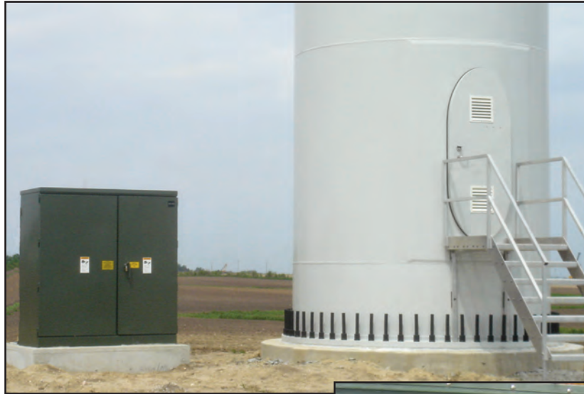
▲ Padmount switch installed outside the tower.
