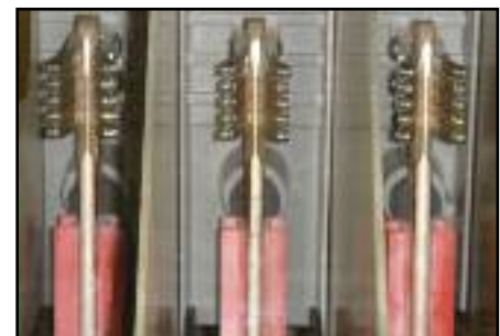
Photos (top to bottom) show closed, ► open and ground contacts as seen through the viewing window.
