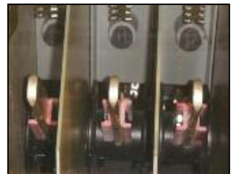
▲ Color coded temperature compensated pressure gauge and fill valve.
