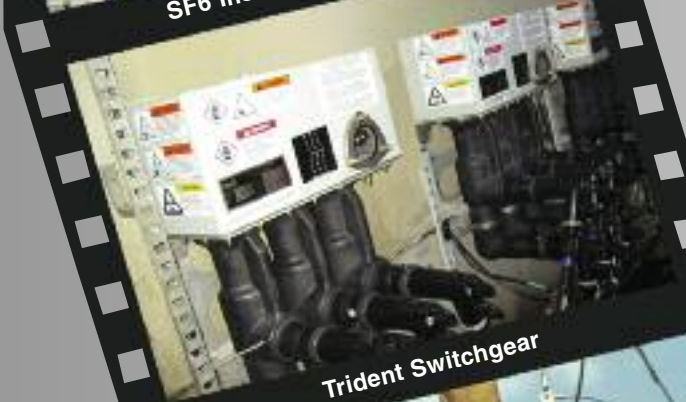
SF6 Insulated Switchgear
