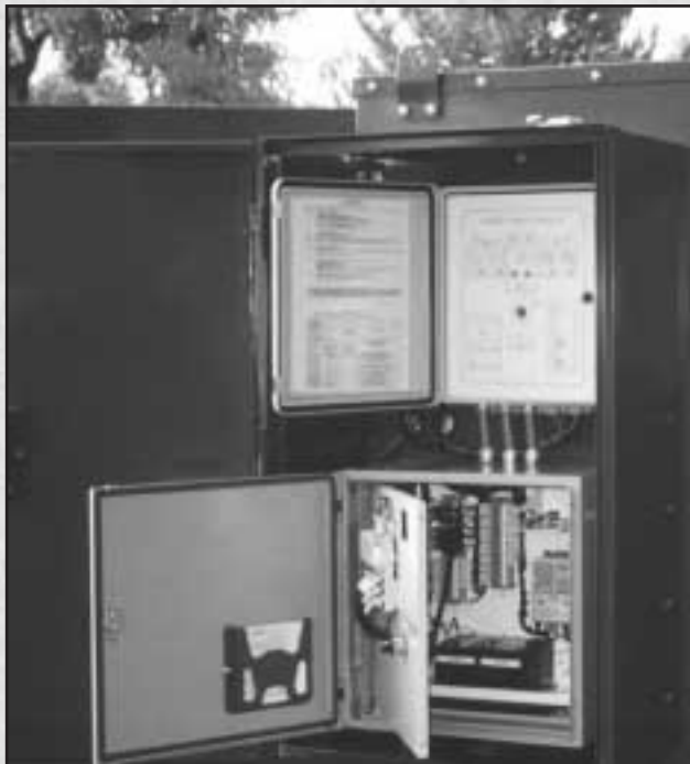
Automatic transfer controls can be combined with RTUs for remote SCADA applications.
