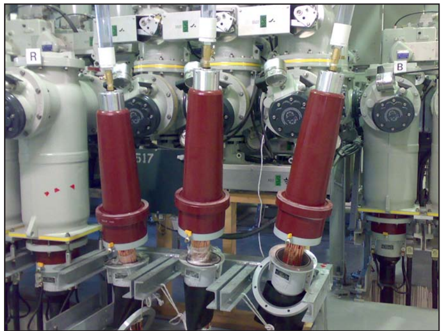
▲ 145kV terminations being prepared for installation in a gas insulated substation
