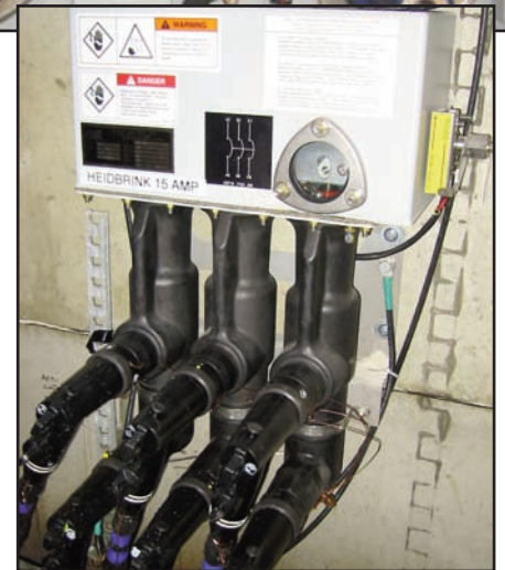
▲ Voltage sensing bushings mounted on a padmount SF6 switch.
