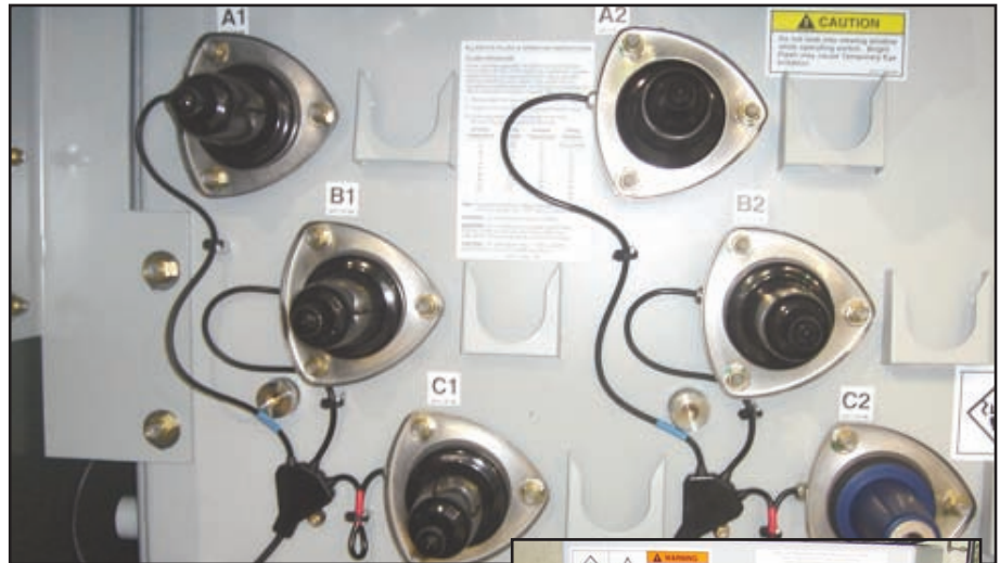
▲ Voltage sensing bushings mounted on a padmount SF6 switch.
