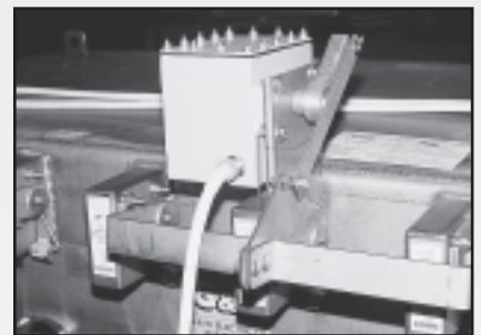
▲ Motor actuators can be added for remote operation.
