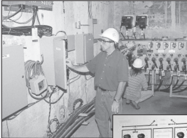
▲ Vault switch application with ATC and RTUs.
