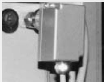
▲ SF 6 density switch
