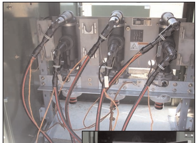
Photo above shows the recloser compartment access for cable connections.
