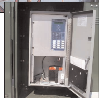
Photo above shows the recloser compartment access for cable connections.
