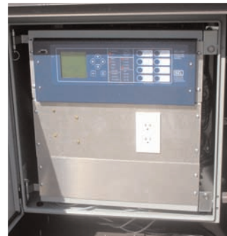
The SEL 451 relay (above) is housed in a separate enclosure on the side of the switch.
