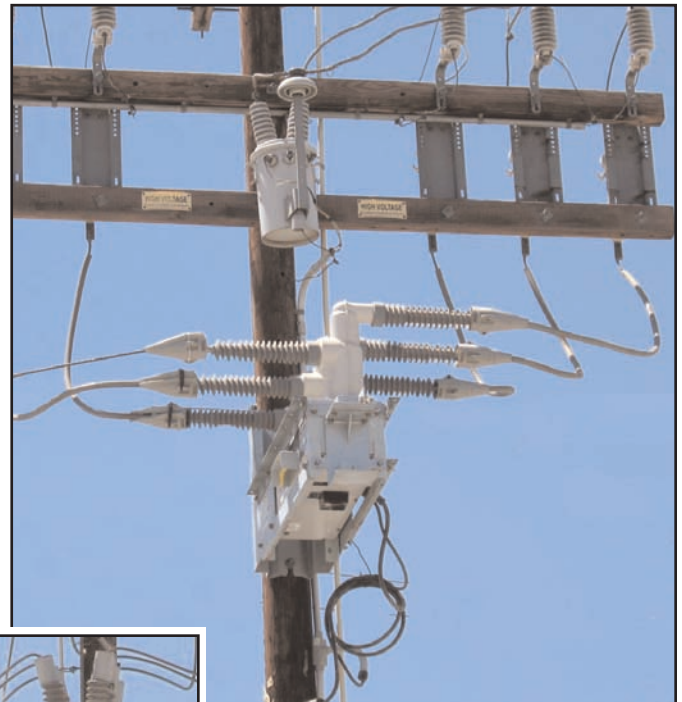
The low profile design of G&W's 38kV recloser (above) permitted maintaining electrical clearances while providing a direct replacement of the old oil-filled gear (15kV shown in inset) without any pole reconstruction.
