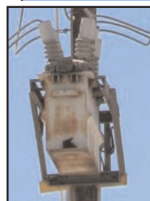
The low profile design of G&W's 38kV recloser (above) permitted maintaining electrical clearances while providing a direct replacement of the old oil-filled gear (15kV shown in inset) without any pole reconstruction.
