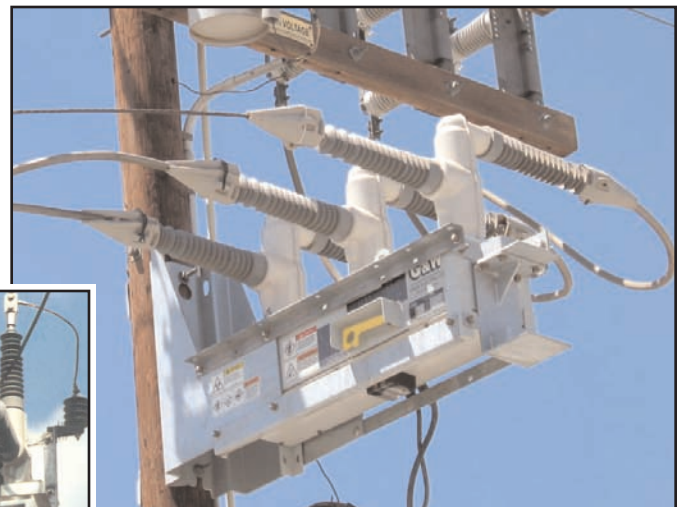
Above: G&W 38kV Viper-S recloser with “Z” modules.
