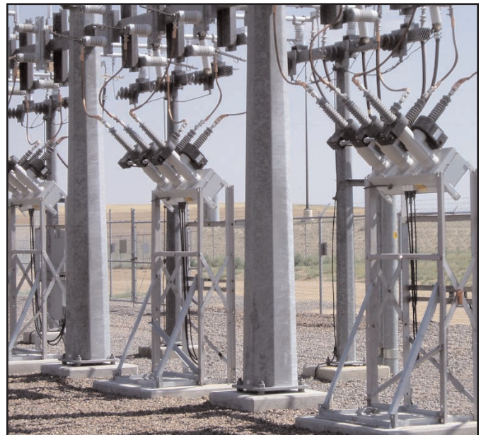
▲ G&W 27kV Viper-S recloser with SEL 351S control.
