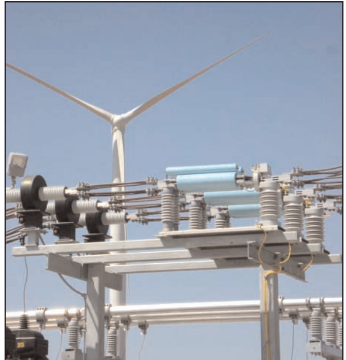
▲ 38kV current limiting protectors mounted at the utility grid substation protects the utility from potential wind farm faults and the wind farm from potential utility faults.
