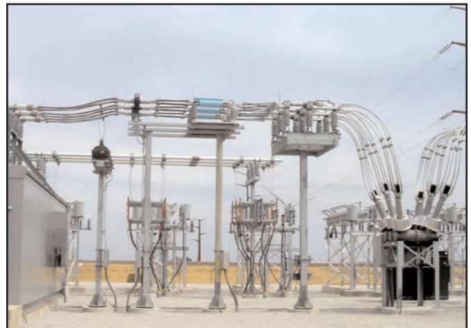
▲ 38kV current limiting protectors mounted at the utility grid substation protects the utility from potential wind farm faults and the wind farm from potential utility faults.
