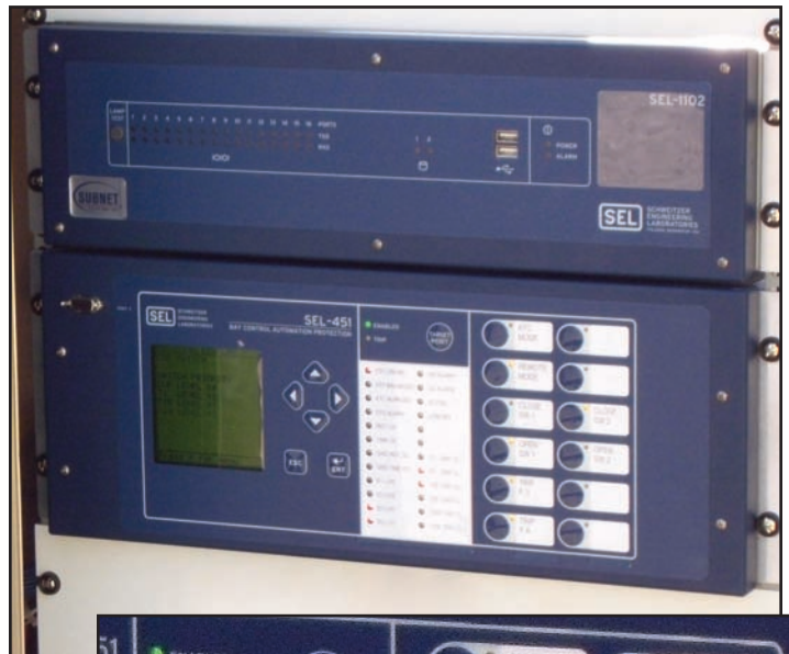
The SEL 1102 central processing unit is mounted within one of the SEL 451 relay cabinets on the side of the switch.
