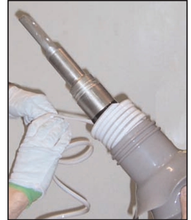
▲ Mechanical shrink installation
