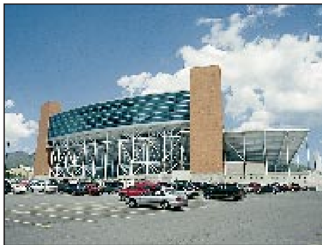
Fig. 3. Completed expansion of the stadium.
