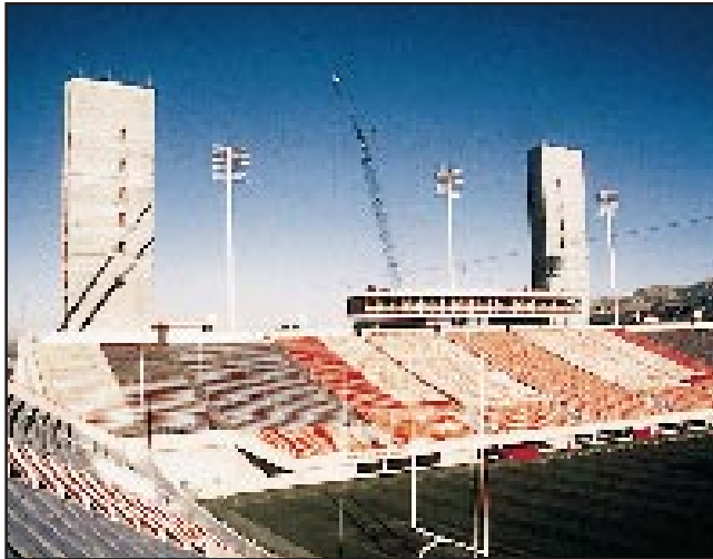
Fig. 2. Rice Stadium under construction.
