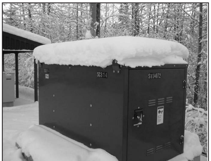
▲ Padmount Viper recloser in a subzero application.
