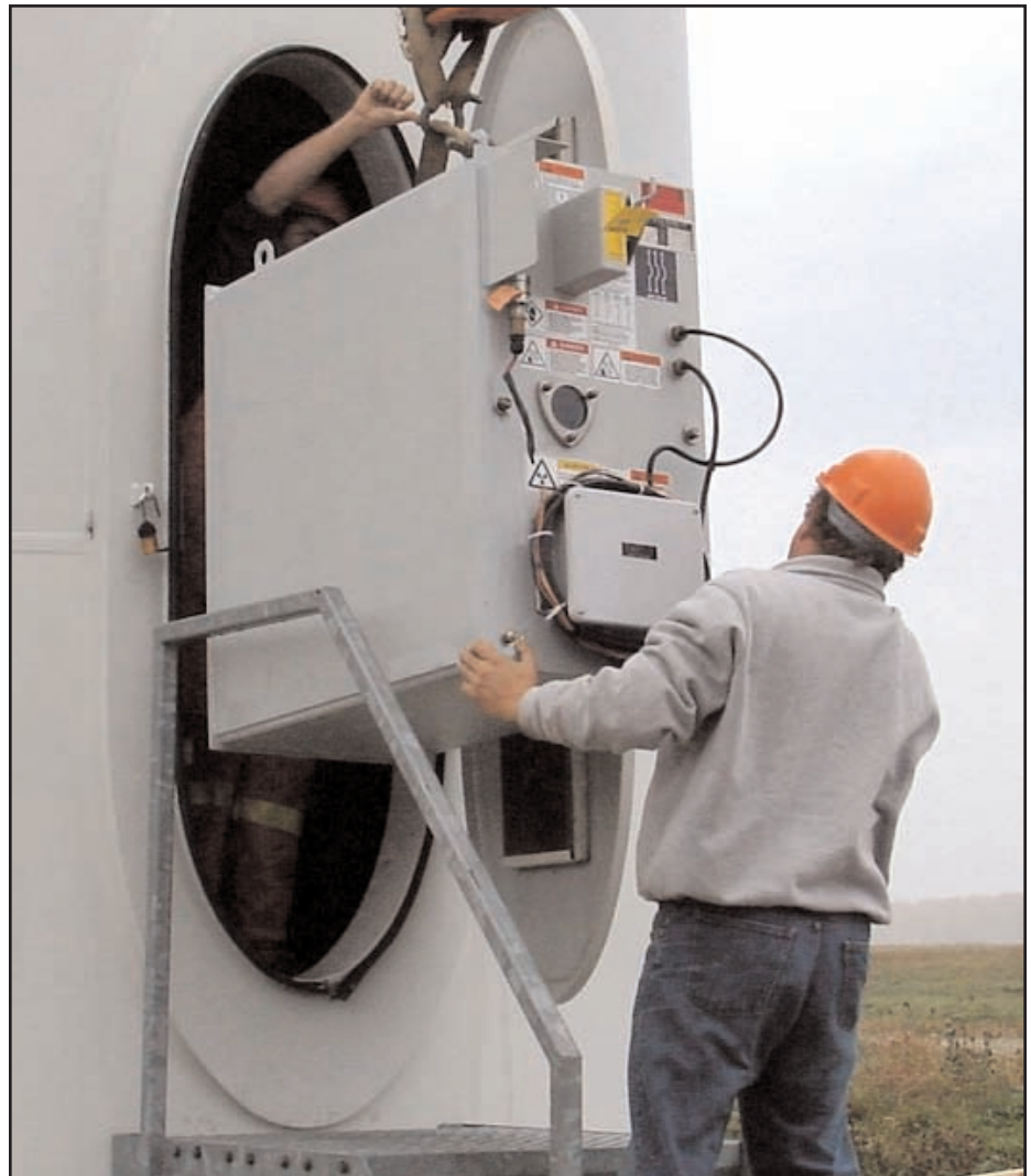
▲ Compact vertical design fits through the typical entrance opening for installation after the tower is constructed.
