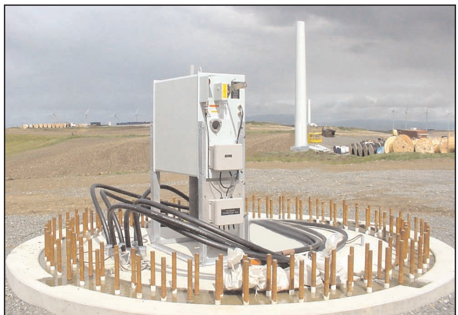
▲ Compact vertical design fits through the typical entrance opening for installation after the tower is constructed.
