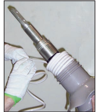
▲ Mechanical shrink installation
