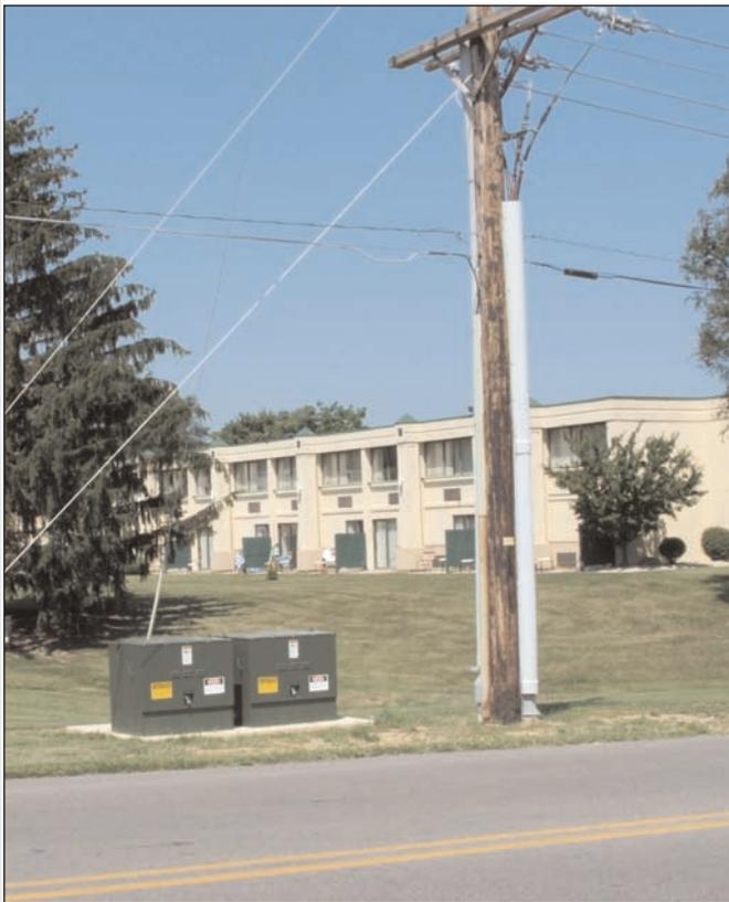
Each of two separate circuits were terminated into padmount enclosures located adjacent to each other.
