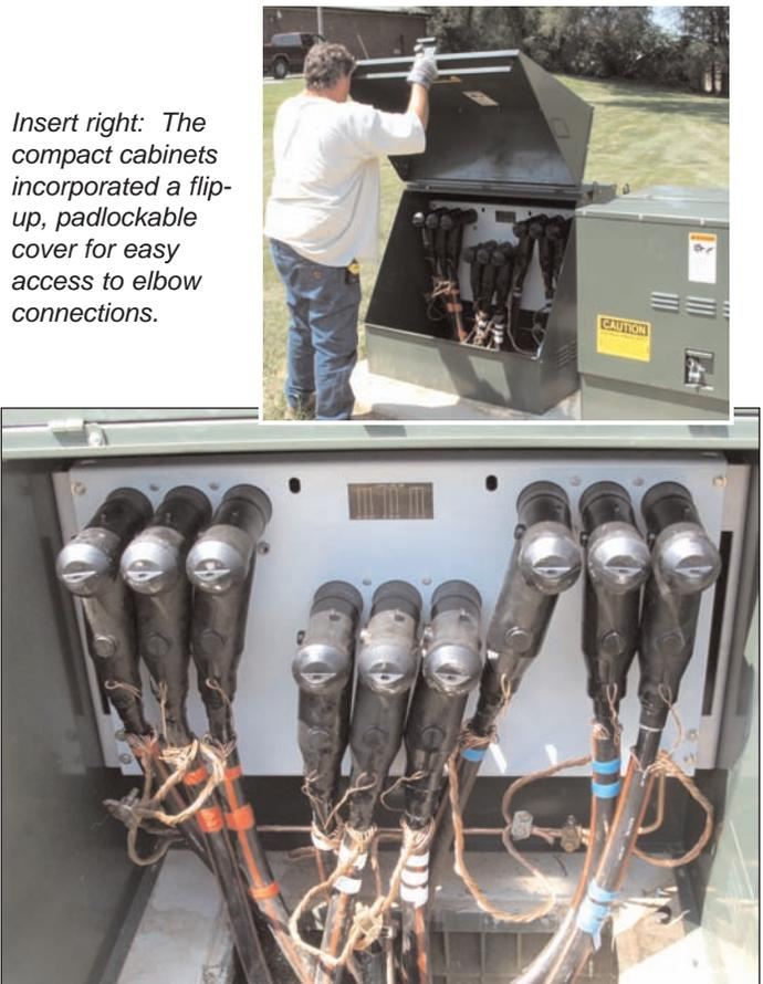
Insert right: The compact cabinets incorporated a flip-up, padlockable cover for easy access to elbow connections.
