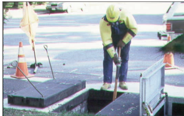
▲ Subsurface vault switches can be hookstick operable from above ground.
