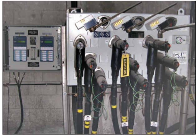
▲ Three-way vault switch with control.
