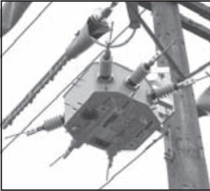
G&W's overhead Linear Puffer (LP) load break switches are designed for operation on distribution systems rated through 38kV, 630A continuous and 40kA asymmetrical short circuit. LP switches can accommodate almost every user switching requirement. The switches are designed and tested to applicable ANSI and IEC standards.
