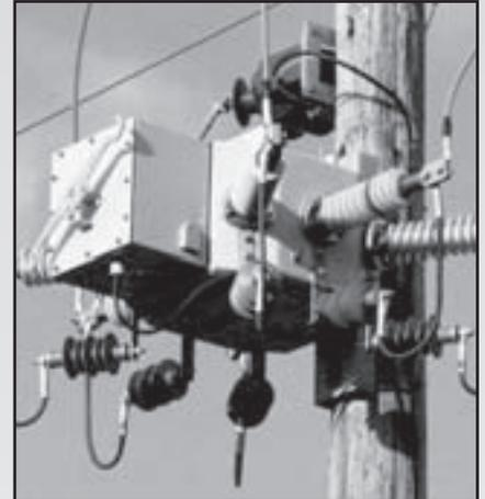
▲ *RP style switch with motor actuator.*
