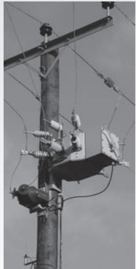
▲ *15kV, model RP switch with lightning arresters and potential transformers.*
