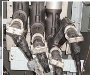
*Insert left: Shows the outer phase PT connection using a dead-front "H" connector on the switch.*
