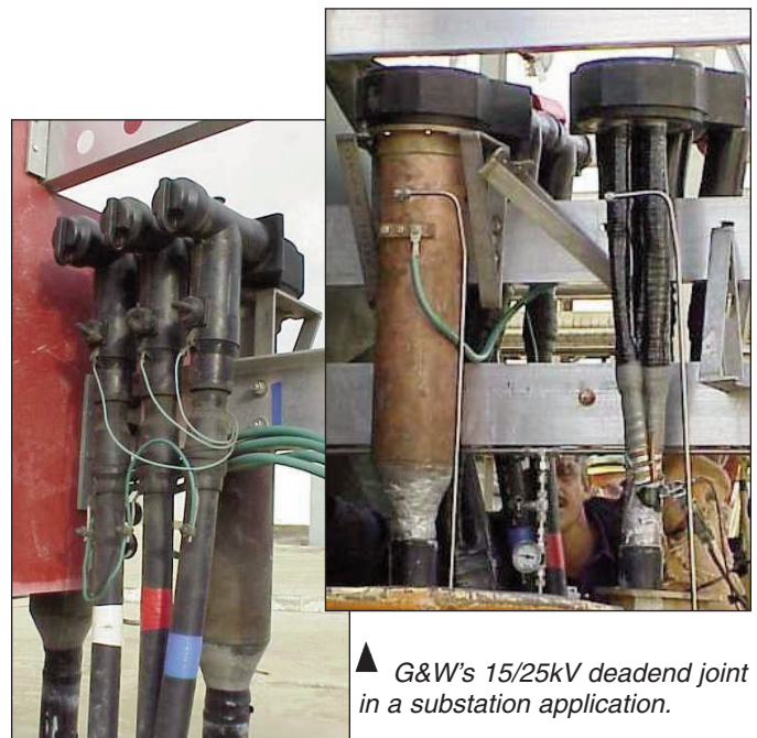
▲ G&W's 15/25kV deadend joint in a vault application.
