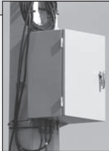
▲ 15kV model RP switch with lightning arresters and potential transformers.
