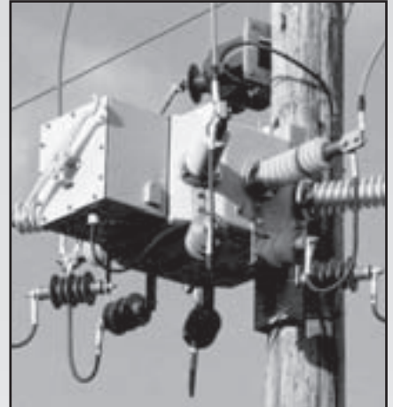
▲ RP style switch with motor actuator.
