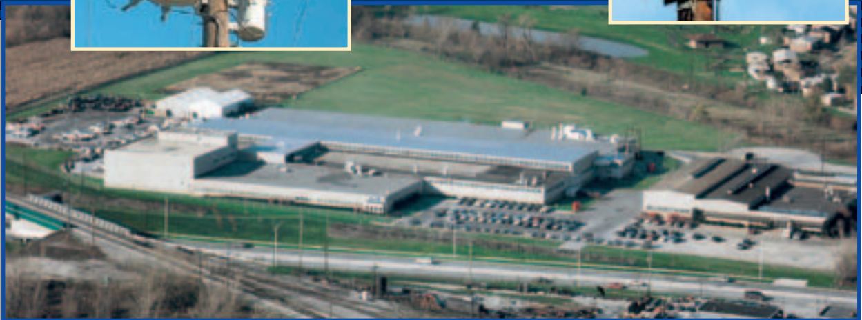
G&W Electric headquarters located in Blue Island, Illinois USA.
